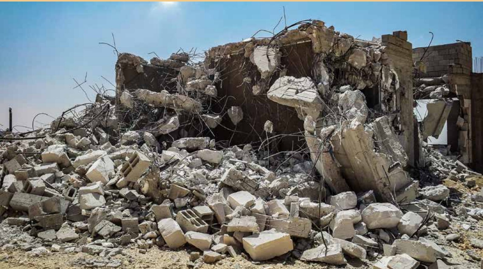
Above: The remains of Bassam Ibrahim's demolished house. Photograph sourced from the Al-Marsad archives.
